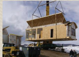
Modular components are placed using a crane. Components are built inside avoiding harsh winter conditions
